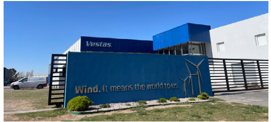
Vestas training and warehouse center - Bahía Blanca
